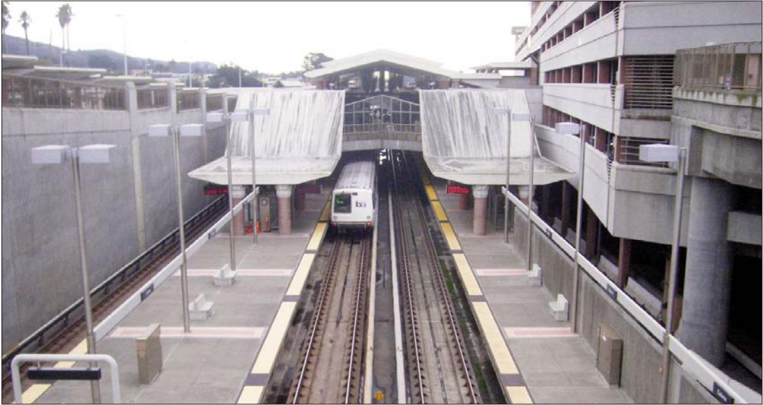
View of the platforms from bridge to parking structure. The parking structure is to the right.
