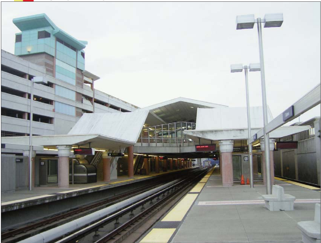
View from the platform level looking toward the concourse. The parking structure is to the left.
