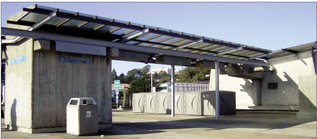
The entrance to BART from Geneva Avenue.
