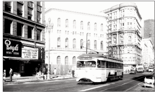
Market Street at Powell Street in San Francisco during the construction of the BART tunnel, ca. 1971, see pages 38-39.see pages 48-49.
