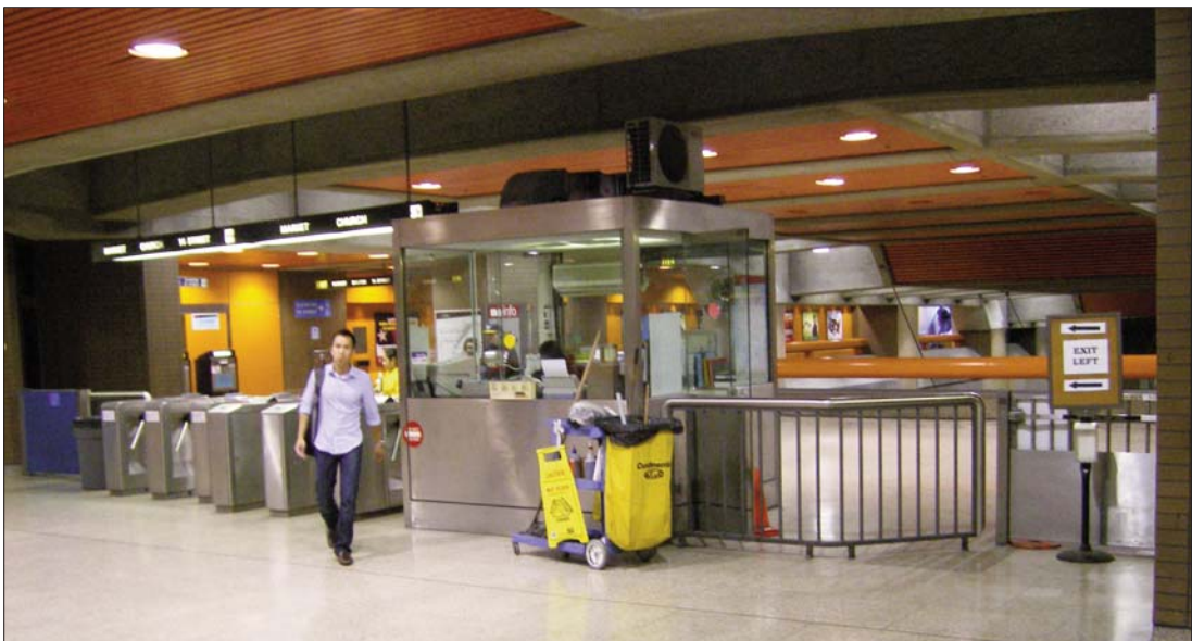
Entry barriers and station agent's booth, mezzanine level.
